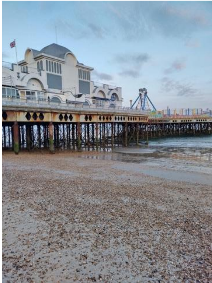
Photograph Z.2b.3 : South Parade Pier from the Beach
