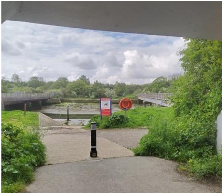
Photo Z7.2: PRE & Signage at Highbury Motorway Underpass
